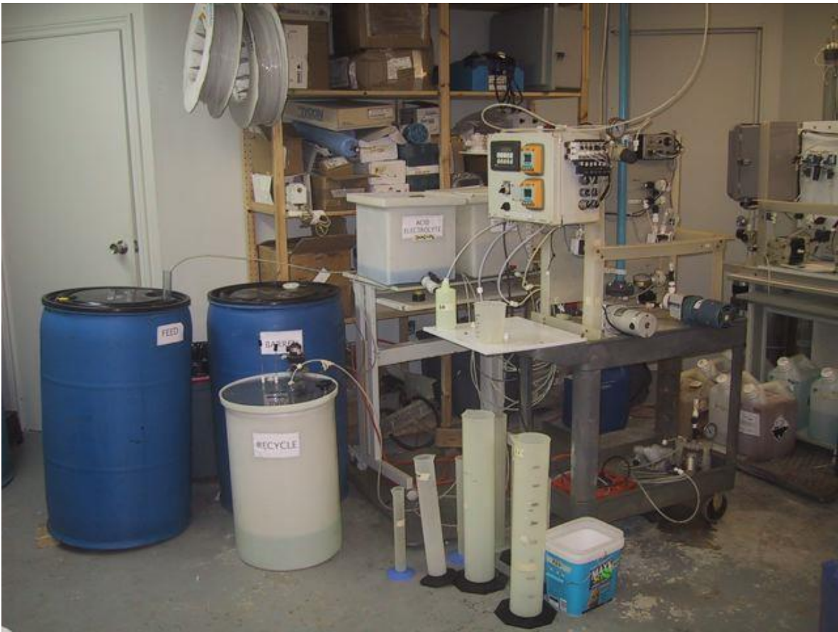
Figure 1: IX Pilot Plant Set-up
